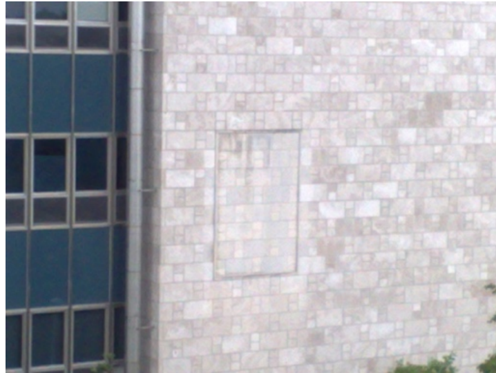
Fig. 2. View of inspected wall.
