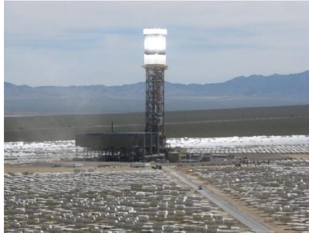
Fig 1. Power Tower during Operation
