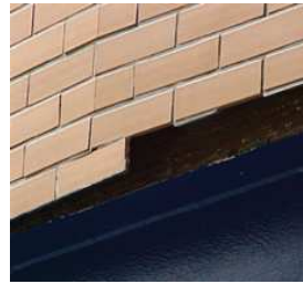
Fig. 2. Detachment of ceramic tiling.
