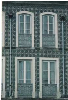
Fig. 1. Portuguese ceramic cladding façade.
