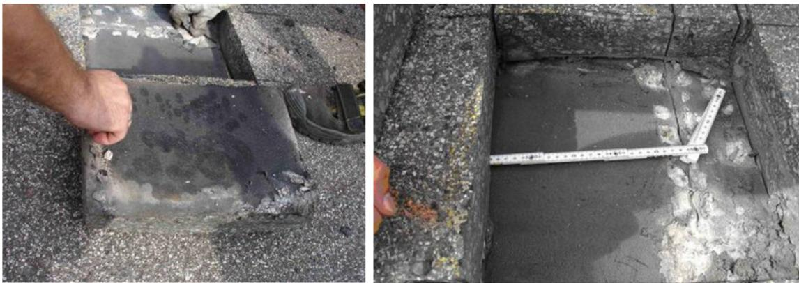
**Fig. 4.** Opened damaged spot, detected by IR-image before (figure 1); lack of bonding demonstrated by means of a ruler.
